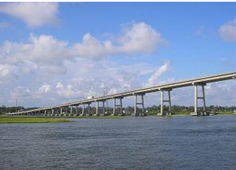
B. Cameron Langston Bridge (0.9 mi long, 65 ft high)
