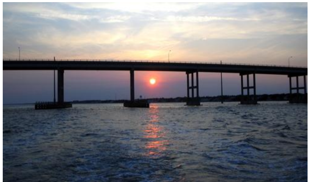
Atlantic Beach – Morehead City Bridge (bike friendly design, 0.75 mi)
