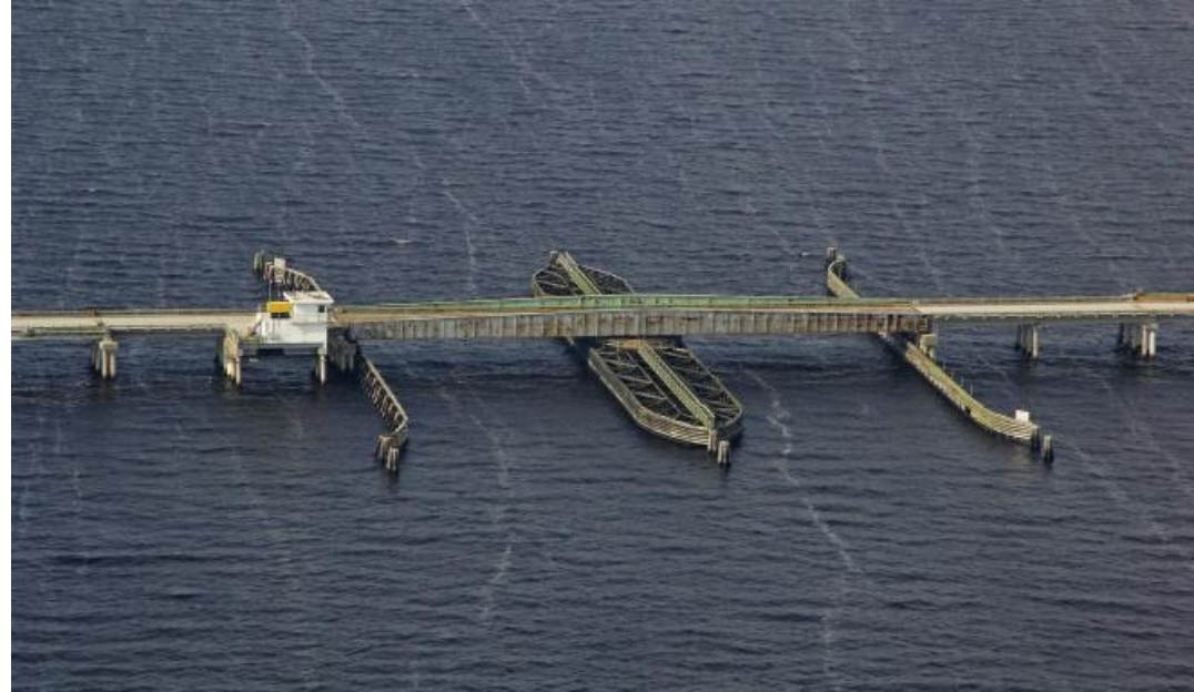
Lindsay Warren Bridge over Alligator River (2.8 mi)
