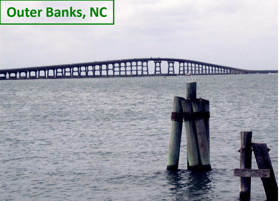
Bonner Bridge over Oregon Inlet (2.5 mi)
